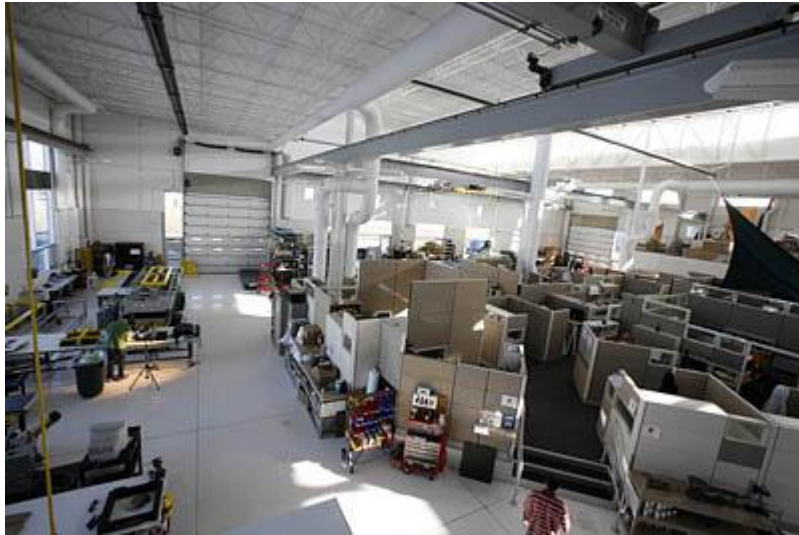
The Radius Engineering building was designed to be energy efficient as well as employee-friendly, employing things such as more efficient heating, cooling, lighting and use of space. The manufacturing area is not far from the office space, but is not crowded and is lit by indirect lighting with large windows.
